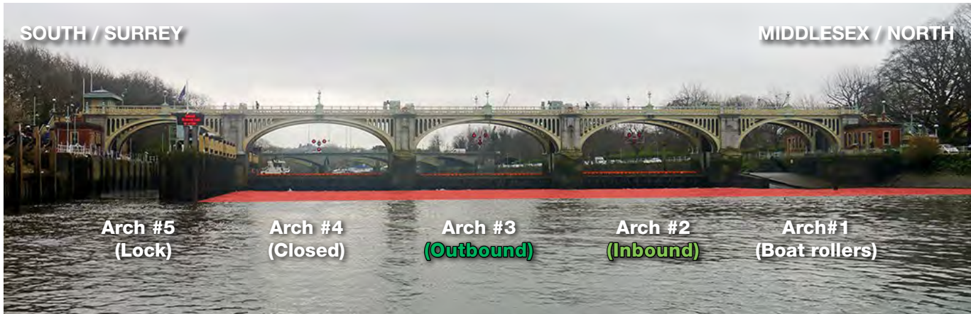
Above: Looking upriver from below the weir, showing the barriers down
